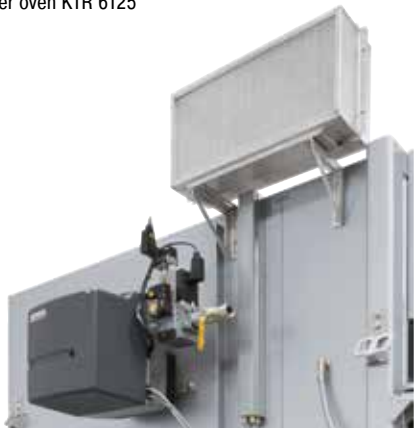
Direct gas-firing at a chamber oven
